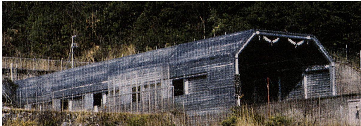
Figure 6: Tunnel hood (49 m long).
